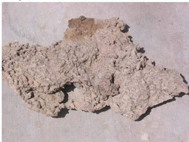
Figure 5 Silica scaling sample removed from a steam pipeline at Cerro Prieto geothermal field
