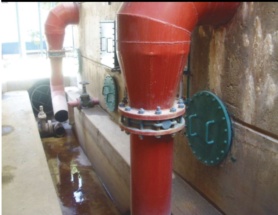
Coatings for protection against corrosion pipelines.
